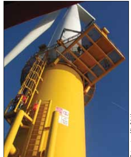
The wind turbine monopile – galvanic anodes were installed inside the sealed portion of the monopile below the lower platform.
