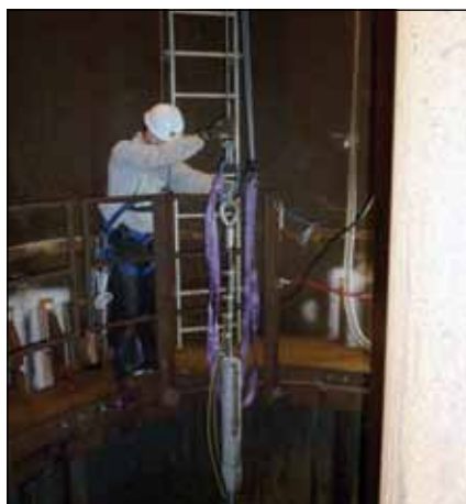
Above left and centre: A trial anode string is lowered into the monopile's contained water.
