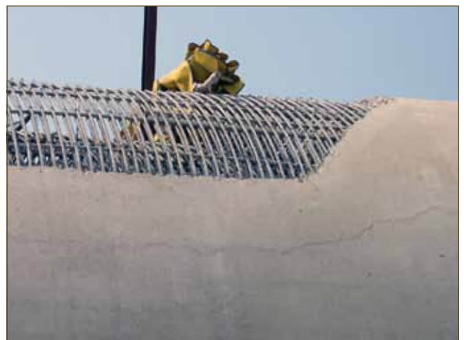
Changi outfall pipes, Singapore.
