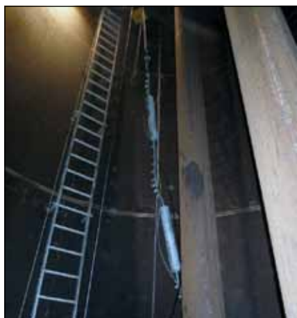
Above left and centre: A trial anode string is lowered into the monopile's contained water.
