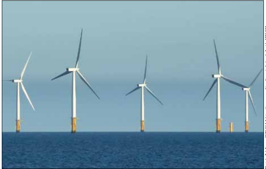
Lynn and Inner Dowsing is a combination of two wind farms located off United Kingdom's East Lincolnshire coastline in the North Sea.
