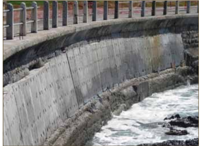
Cape Town seawall, South Africa.
