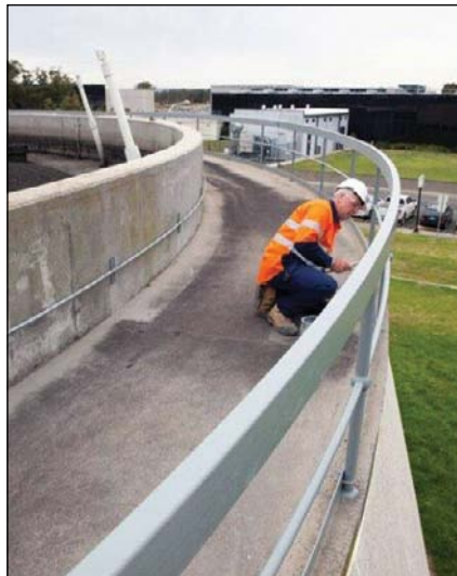
Protecting the metalwork around a water storage facility.
