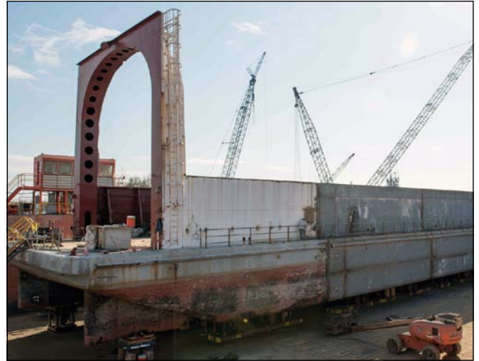
Surface preparation and repairs underway on Pegasus barge, which will ship rocket components for deep space missions. (Source: NASA/Steven Seipel)
