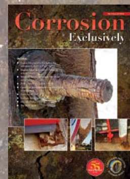
Cover: A collage of corroded components at the coast.
