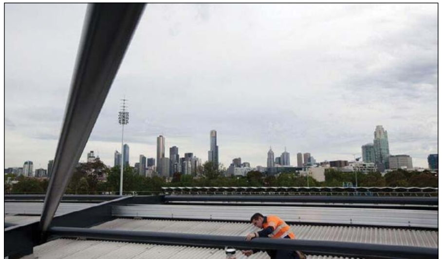
Applying a protective coating to the roof of a sports complex.
