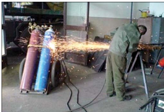
Work place hazards.
