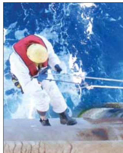
Technician abseiling down the support structure of an offshore rig.
