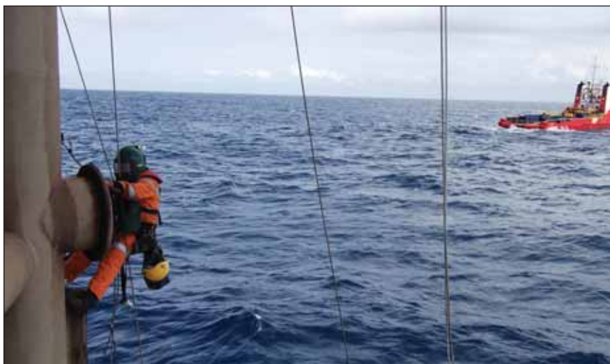
Technician and support ship with an offshore structure.
