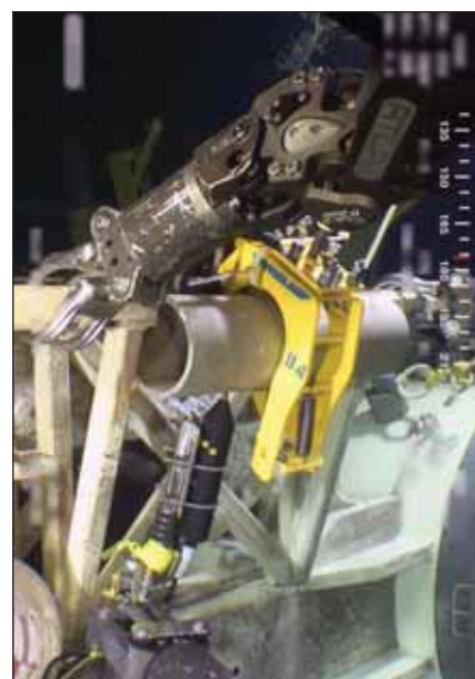
Clamping an anode to an underwater pipeline.
