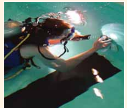
The author, years after the story described here, carries out an underwater repair coating application on one of the highest swimming pools in the world in a skyscraper in downtown Chicago.
